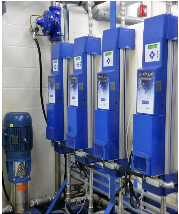
*Four UV Pure Upstream systems provide a high level of disinfection for harvested rainwater, even when UVT is as low as 60%.*
