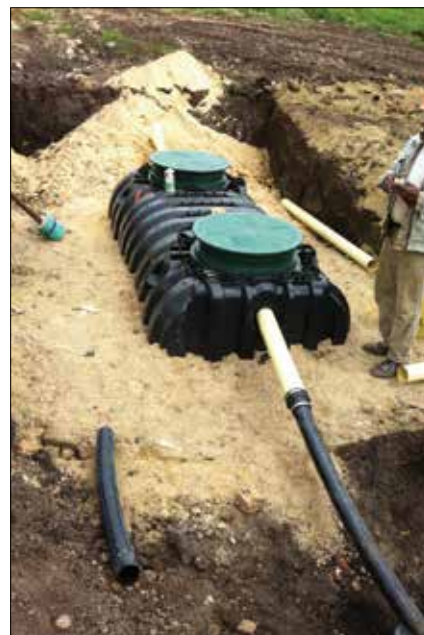
Figure 5 – Installation of an interceptor tank at a new development in Colombia.
