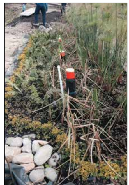
Figure 6 – Construction of a modular horizontal flow constructed wetland in Colombia
