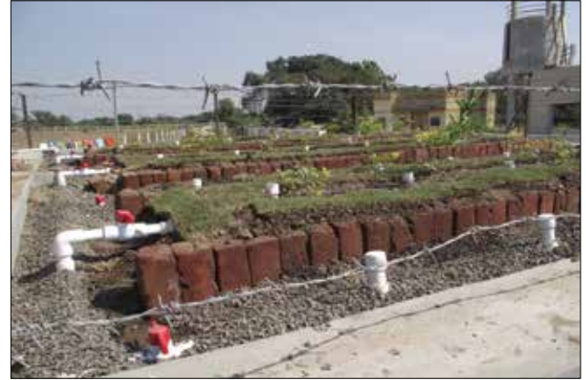
Figure 4 – Vertical flow constructed wetland at a rural village in India.
