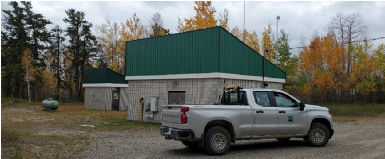
PICTURED 4: PICKLE LAKE WATER TREATMENT PLANT
