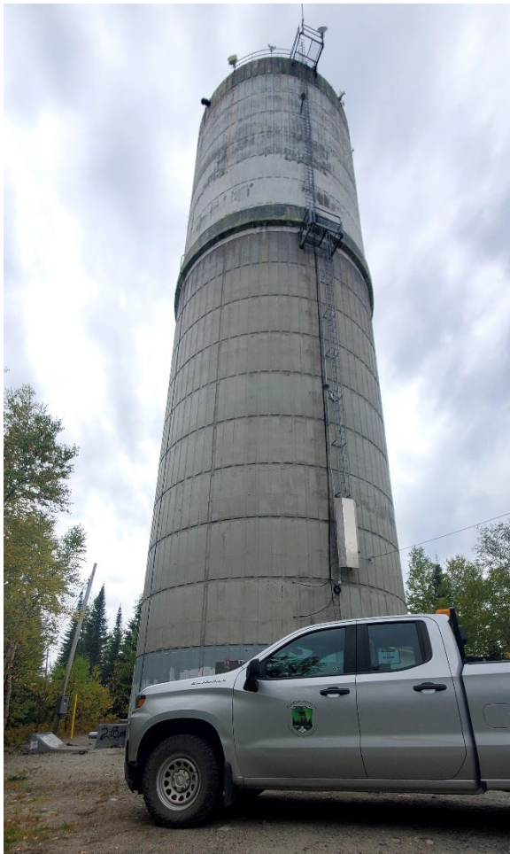
PICTURED 2: WATER TOWER FOR THE PICKLE LAKE TOWNSHIP
