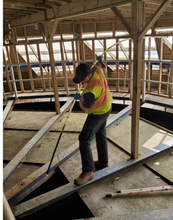
PICTURED 3: MEASURING THE CLARIFIER SLUDGE DEPTH
